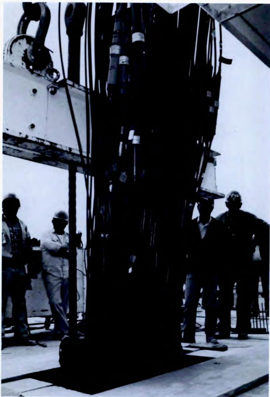
View of surface Ground Zero during the emplacement operation showing emplacement hardware and diagnostic cable bundle that connects the downhole equipment with the recording trailers. The small cylinders on the cables are gas blocks that prevent the flow of downhole gases through the cables to the atmosphere.
